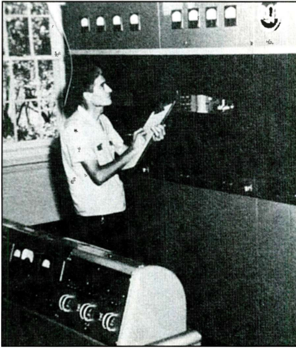
WXXW's Mike Capri logs a reading from the station's big 10-kW RCA transmitter. Figures from its related antenna phasing equipment were the numbers management most dreaded.
